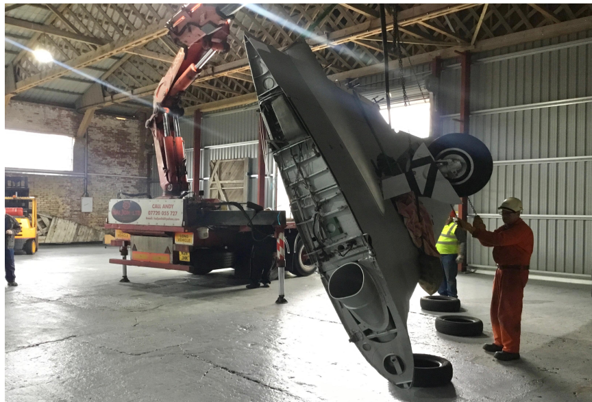
Lifting the Vampire's wings into position.
